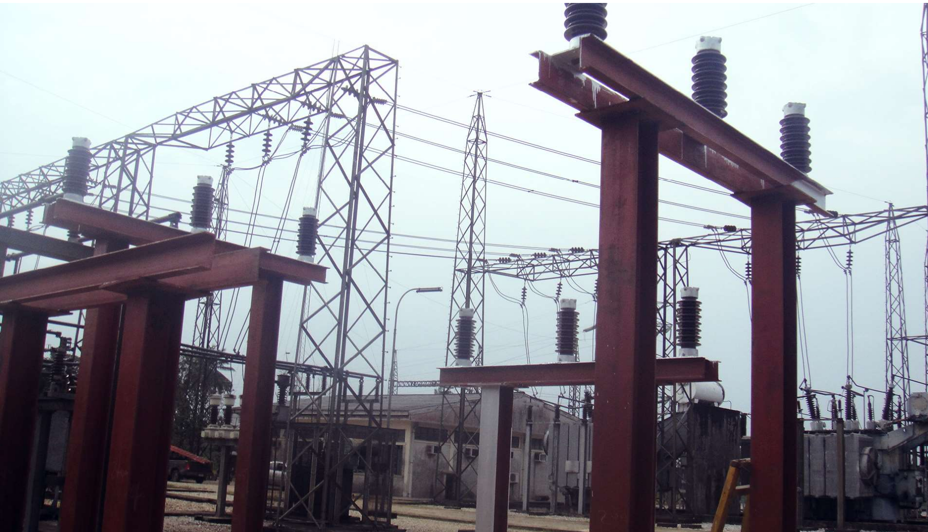
33KV Feeder Bays at EKET Substation
