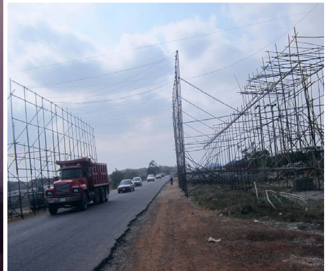
Lot 3 Project Cable Laying Cross The Road
