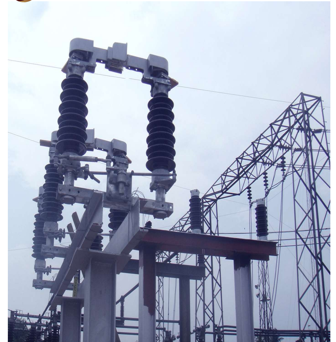
33KV Feeder Bays at EKET Substation
