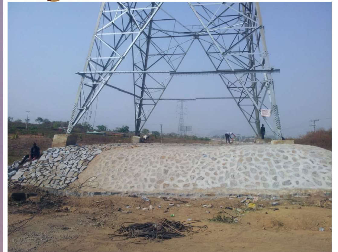
Lot 3 Project Foundation And Stone Oitching For Tower
